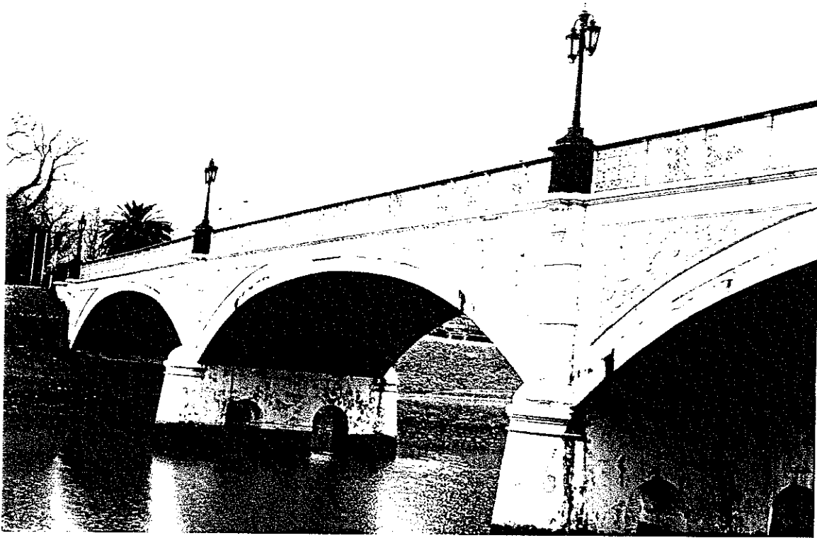
Photograph 1: Condition of Morell Bridge before restoration
